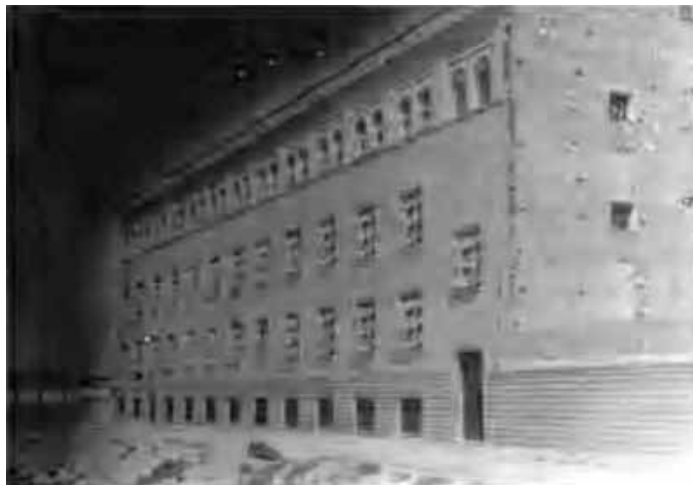
Fachada principal (sin terminar)
